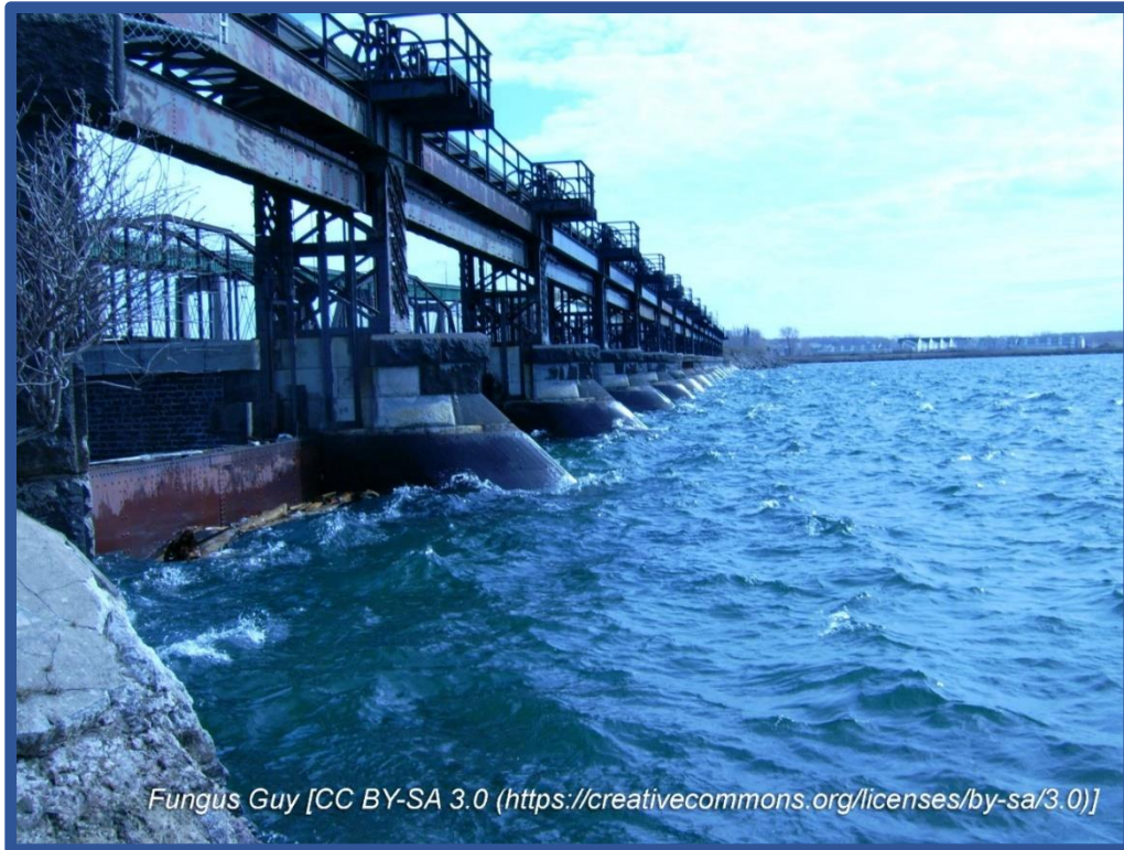
The Compensating Works regulate flow from Lake Superior to Lake Huron.
