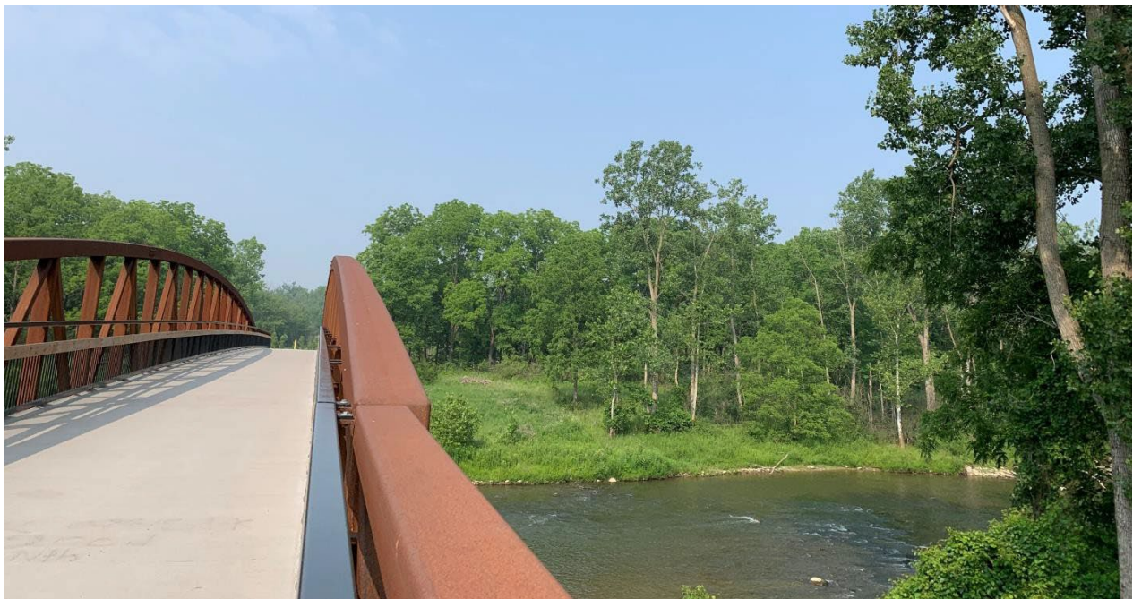
New foot bridges were installed over the north Thames River in London in 2021 to extend the Thames Valley Parkway multi-use trail. Photo by Cathy Quinlan
