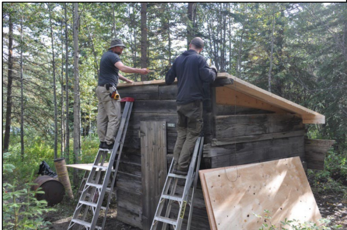
Replacing the roof on an historic building in 2021.
